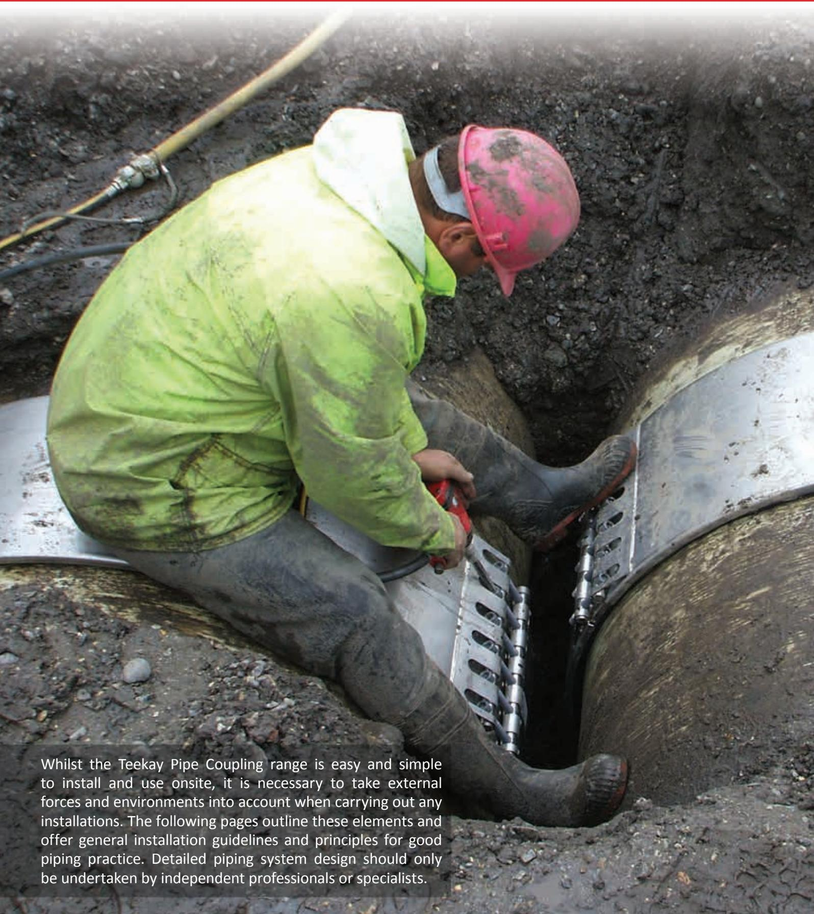
Whilst the Teekay Pipe Coupling range is easy and simple to install and use onsite, it is necessary to take external forces and environments into account when carrying out any installations. The following pages outline these elements and offer general installation guidelines and principles for good piping practice. Detailed piping system design should only be undertaken by independent professionals or specialists.
