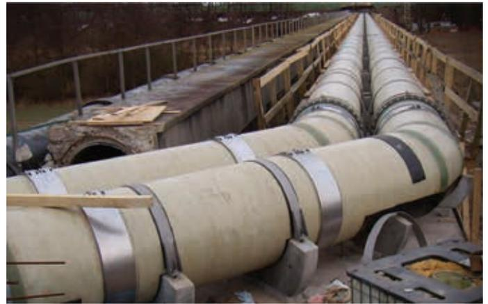
Buried pipelines can generally be restrained by means of thrust blocks at major changes in direction. Straight runs and minor curves are usually restrained by soil friction. The same is largely true of gravity or very low pressure pipelines running along the ground, although with certain thermoplastic piping materials special attention should be given to restraining the forces generated by excessive expansion, contraction and creep.
